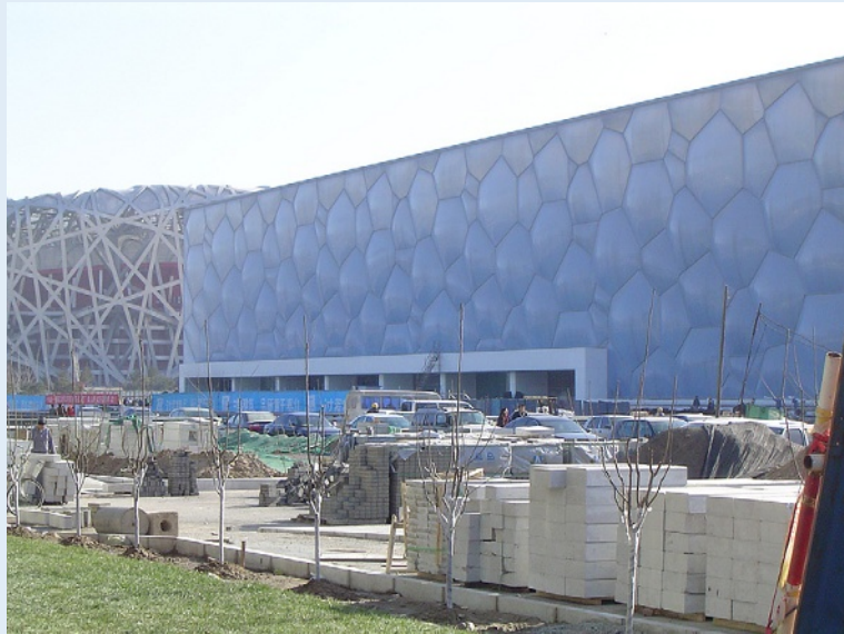
Beijing's new Aquatics Centre, nicknamed the 'Water Cube' nearing completion in late 2007 standing alongside its fellow icon the 'Bird's Nest'.
