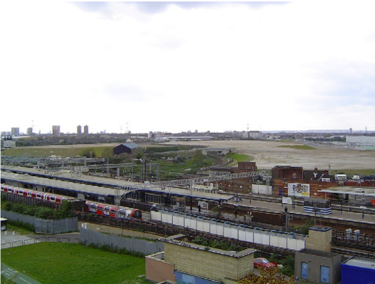
The Olympic Park site for London's 2012 Olympics undergoing early preparation in May 2006.
