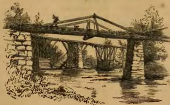
Bridge Across Platte Creek
